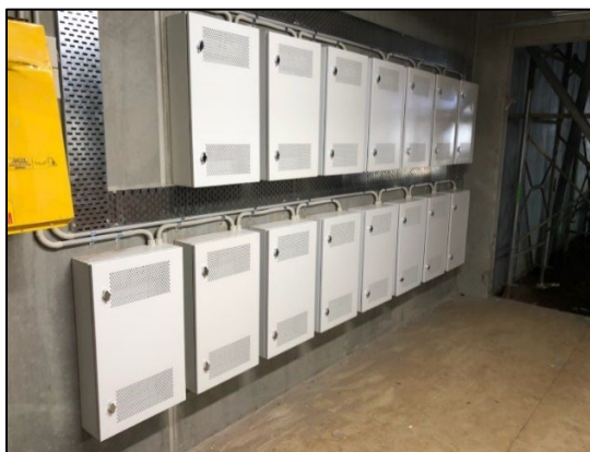
Figure 34. Centrally located NTDs for commercial developments
